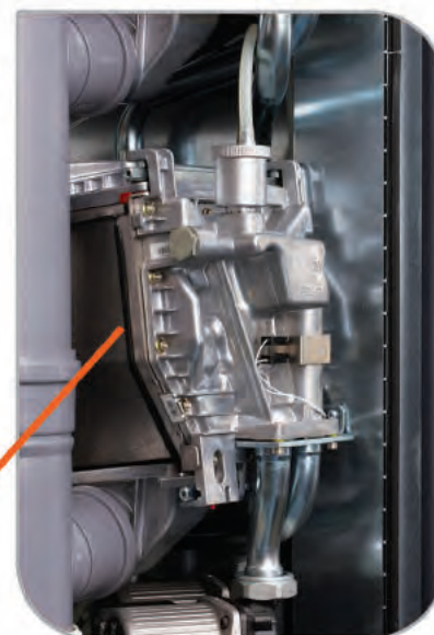
Automatic air vent fitted to highest point of the heat exchanger
